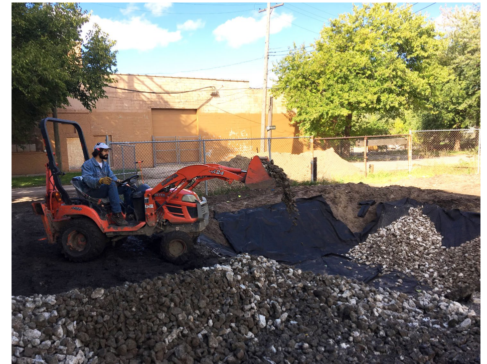
Crew backfilling with small tractor 1
