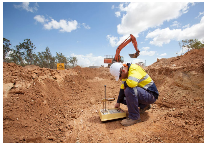
Soil infiltration testing 7
