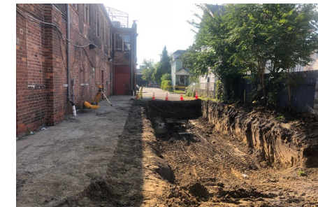
Basin bottom leveled 6
