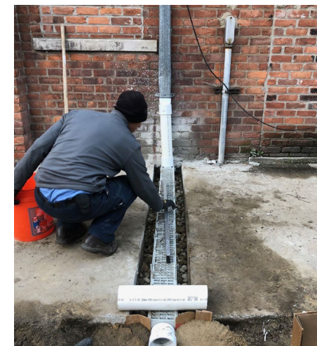
Downspout modified, trench drain installed 1
