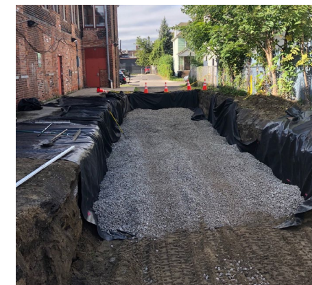
Filter fabric installed, aggregate backfill 7
