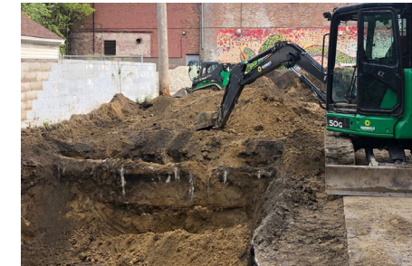
Excavation from the side 5
