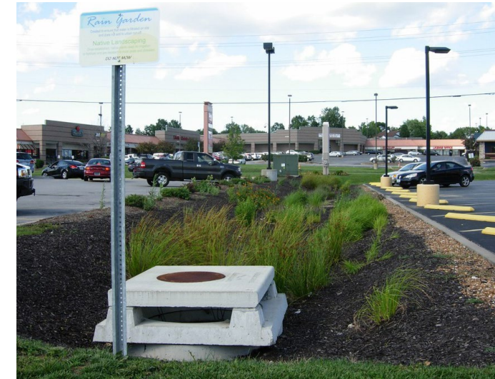
Parking lot bioretention 24
